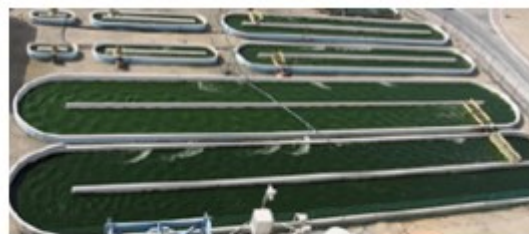
Photo 3-Design of a race-way open pond commonly used for algae culture.
