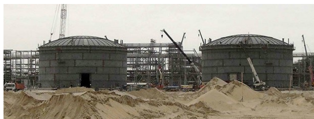
Figure 5 – Sadara 35m Wastewater Tank Construction (3)
