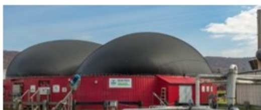
Figure 3 - Anaerobic Digestion (AD) plant
