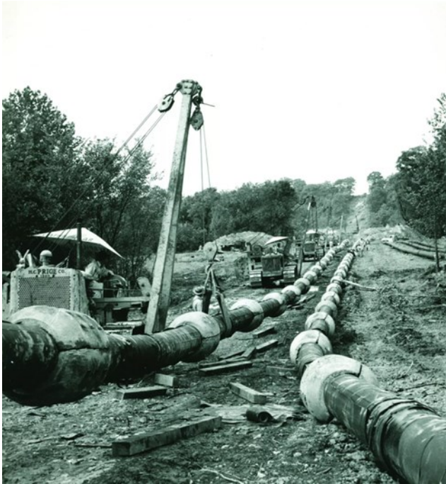
Figure 1. Bolt On Weights on Pipelines [1]
