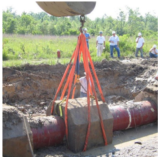
Figure 2. Set On Weights on Pipelines [2]
